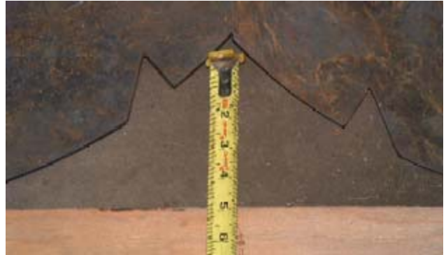
After Installation 5" V
